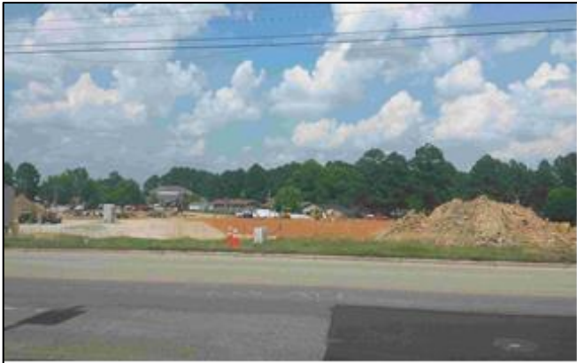
Repetitive Loss Area 7 – Vacant lot under construction
