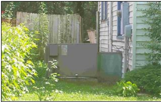
Repetitive Loss Area 10 – HVAC unit on ground
