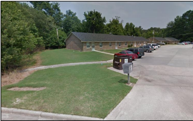
Repetitive Loss Area 17 – Slab-on-grade buildings on fill
