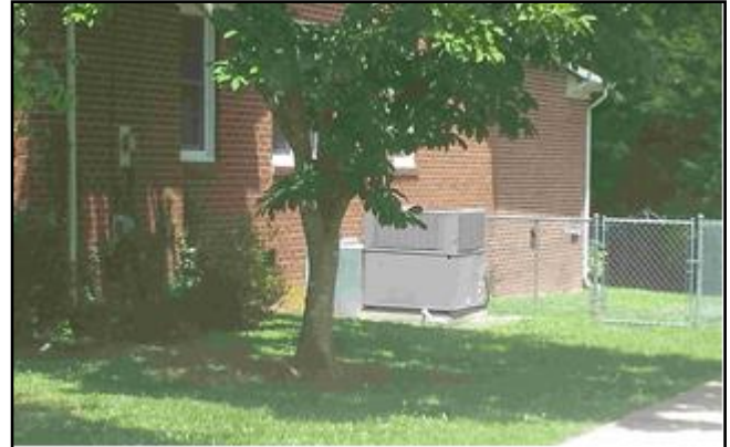
Repetitive Loss Area 3 – HVAC unit on ground
