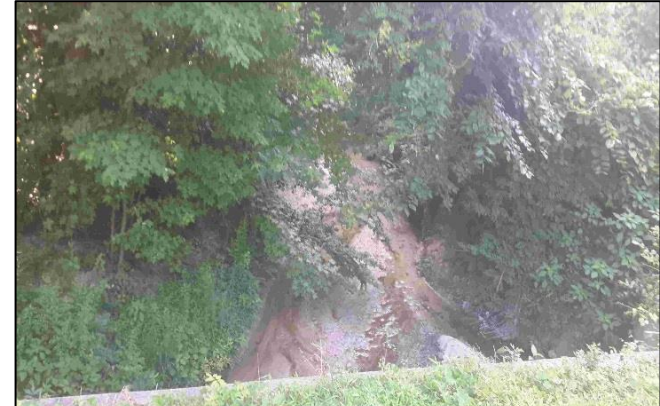
Repetitive Loss Area 8 – Channel adjacent to home
