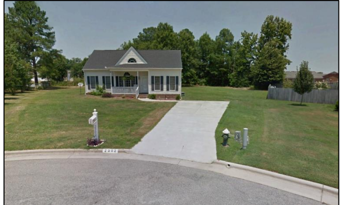
Repetitive Loss Area 16 – Structure elevated on fill; rear yard slopes down to pond
