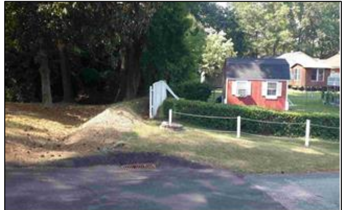
Repetitive Loss Area 12 – Raised berm adjacent to property
