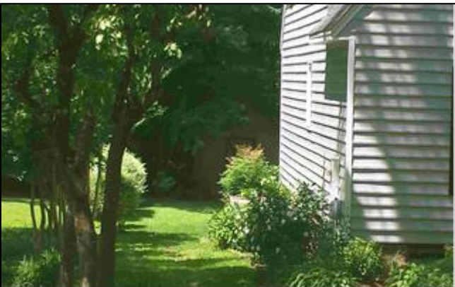
Repetitive Loss Area 6 – HVAC unit on ground
