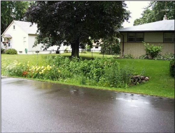
Example of what a rain garden in the right-of-way could look like. Rain gardens capture stormwater, filter out pollutants, and help prevent flooding. Source: lowimpactdevelopmentcenter.org
