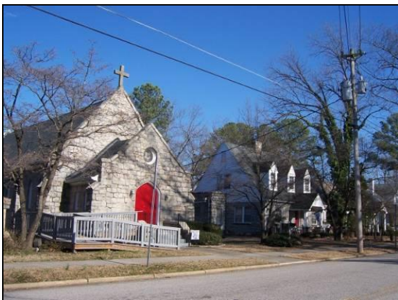
One of the churches in the neighborhood, featuring bellcote form Gothic Revival style architecture.
