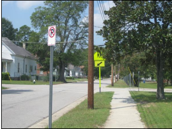
The "parallel" style crosswalk at Margaret Hearne is worn and not very visible from a distance.
