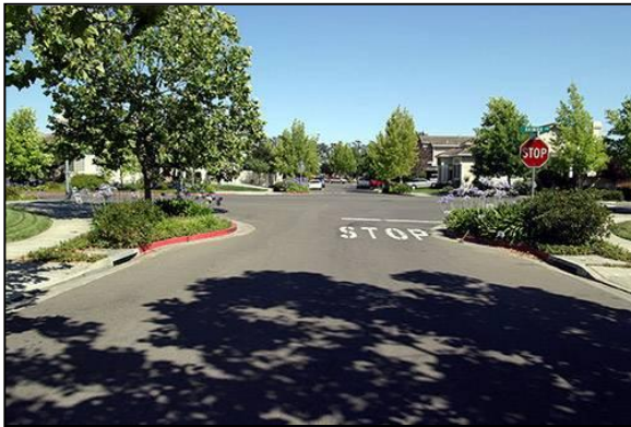
Curb Extensions at intersections (left) or midblock (right) are an example of a possible solution for speeding in the BNO neighborhood. These provide traffic calming that can slow traffic, provide additional landscaping, and help mitigate stormwater flooding. Photo source: www.pedbikeimages.org/ DanBurden
