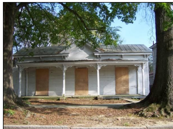
Boarded up structure in the neighborhood.
