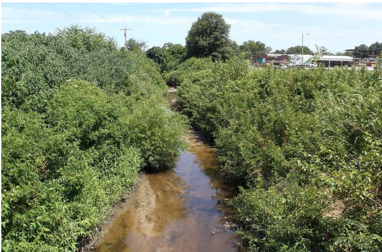
Looking upstream from the Lodge Street bridge towards Goldsboro Street.
