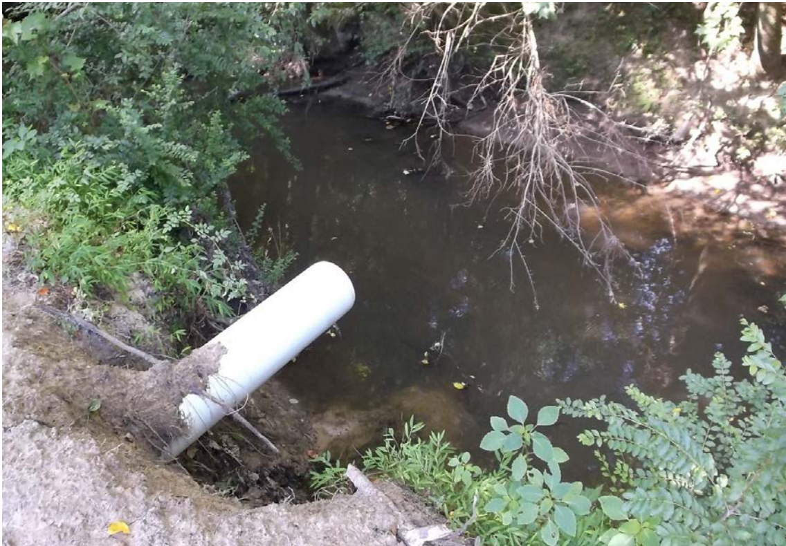
Stormwater outfall from Canal Street emptying into the creek in Reach 2
