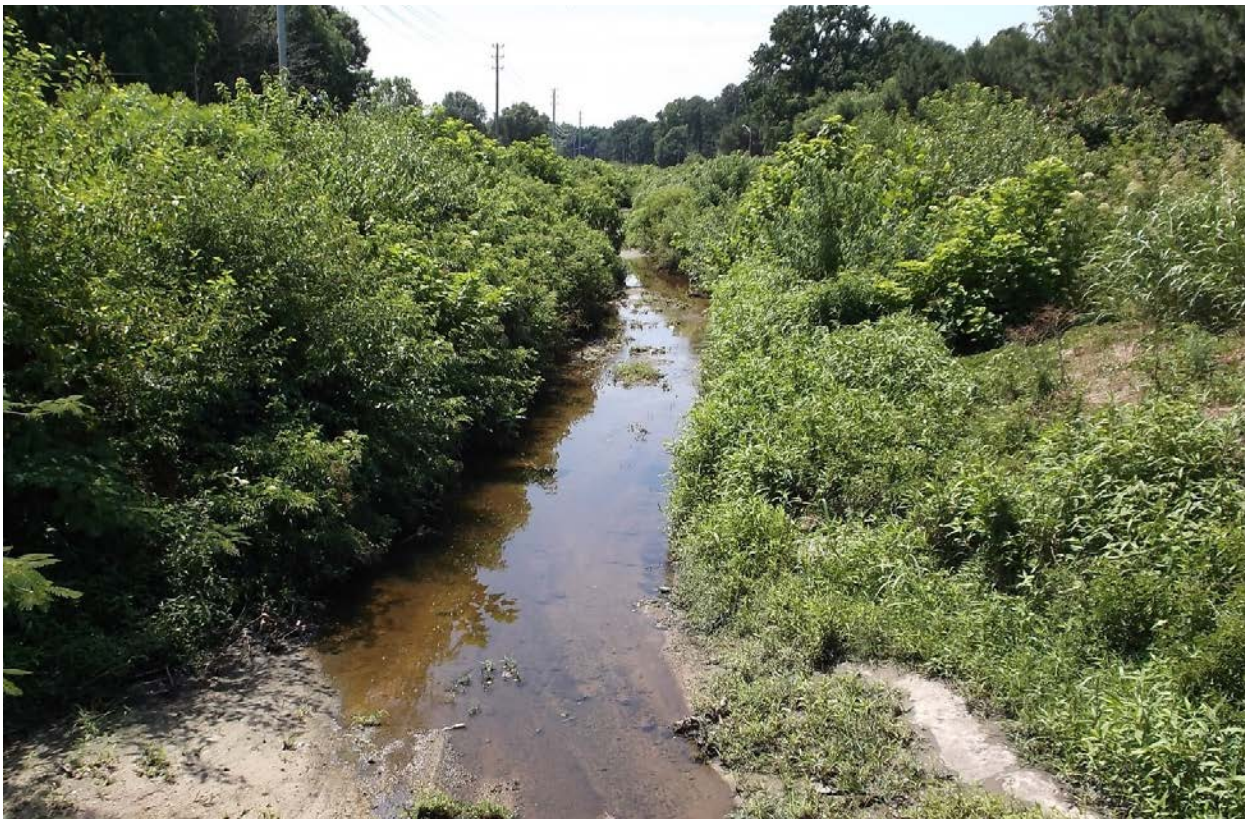
Looking downstream from the Lodge Street bridge.
