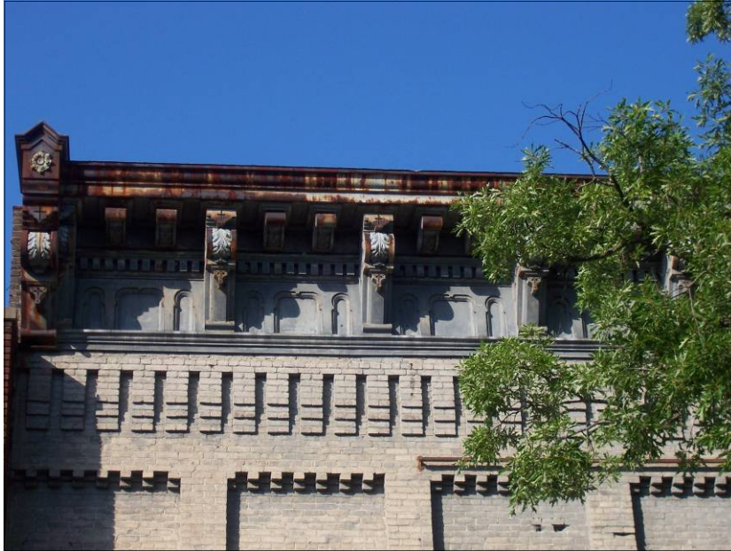
This metal cornice is part of a downtown commercial building and is an example of architectural metal.
