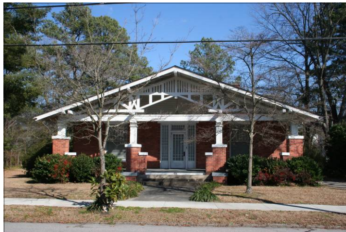
Western Stick Example. Character-defining features include fret-work gable, low-broad roof, Craftsman porch (brick pier with square or tapered posts), exposed beams and rafter tails, and a multiple-pane door flanked by sidelights and transom.
