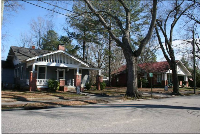
These one-story bungalows are characteristic of the Broad-Kenan Historic District
