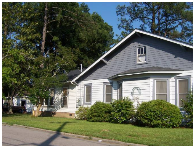
This addition is consistent with the height, scale, size, and proportion of the historic structure.
