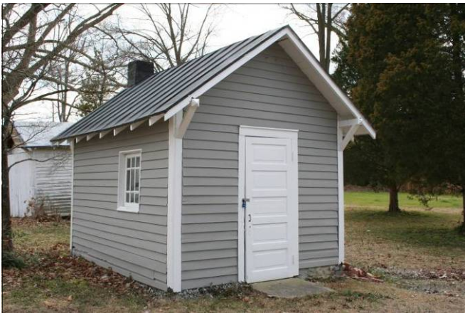
This is a good example of an historic wash house; note the exposed rafter tails, elbow braces, cross-panel door, and standing seam metal roof. All are contributing features to this building.
