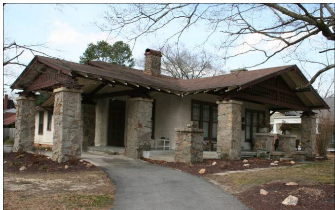
In addition to brick, stone and stucco are masonry materials used in Wilson's historic districts.
