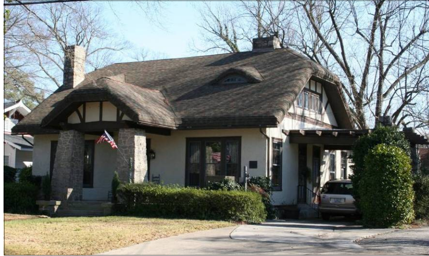
The roof of the Allie Fleming House is a significant, character-defining feature which includes the shingles curving around the roof edge and the eyebrow dormers.
