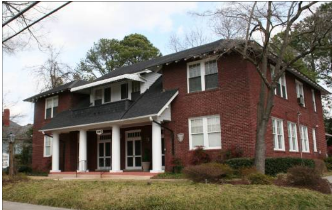
The masonry construction, wide roof overhangs, symmetrical fenestration, and deep porch are all energy efficient elements.
