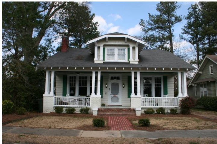
Western Stick Example. Character-defining features include fret-work gable, low-broad roof, Craftsman porch (brick pier with square or tapered posts), exposed beams and rafter tails, and a multiple-pane door flanked by sidelights and transom.
