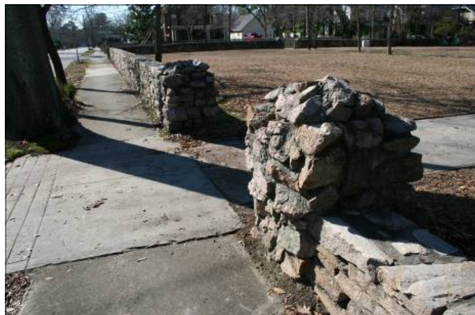
This stone wall is a contributing feature in West Nash.
