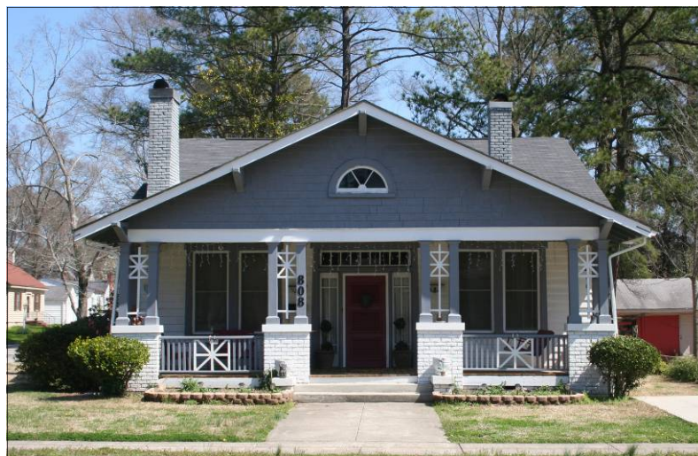
This cross-gable example has an engaged, gable-front porch, brick plinths with paired posts flanking the Smyrna Cross fretwork, a common Wilson feature, central entrance with transom and sidelights, paired windows, wood shingles, and elbow brackets.
