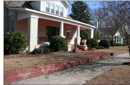
Low retaining walls are common in Wilson's historic districts.
