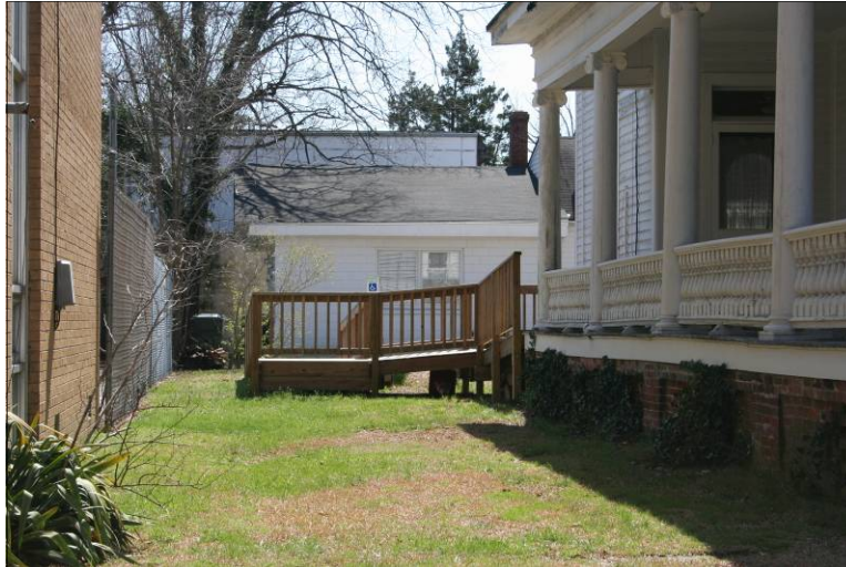
This access ramp is reversible and located on the secondary AVC.
