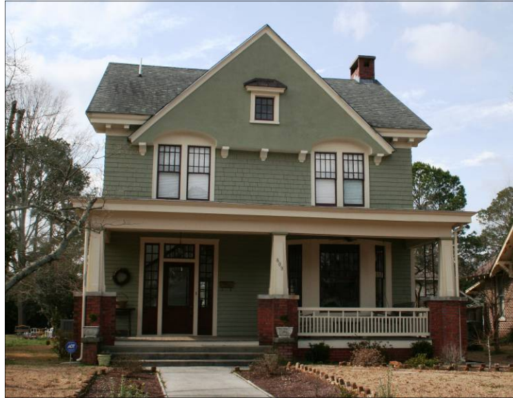
The original wood windows and doors of this house add to the architectural character and visual quality of this home.
