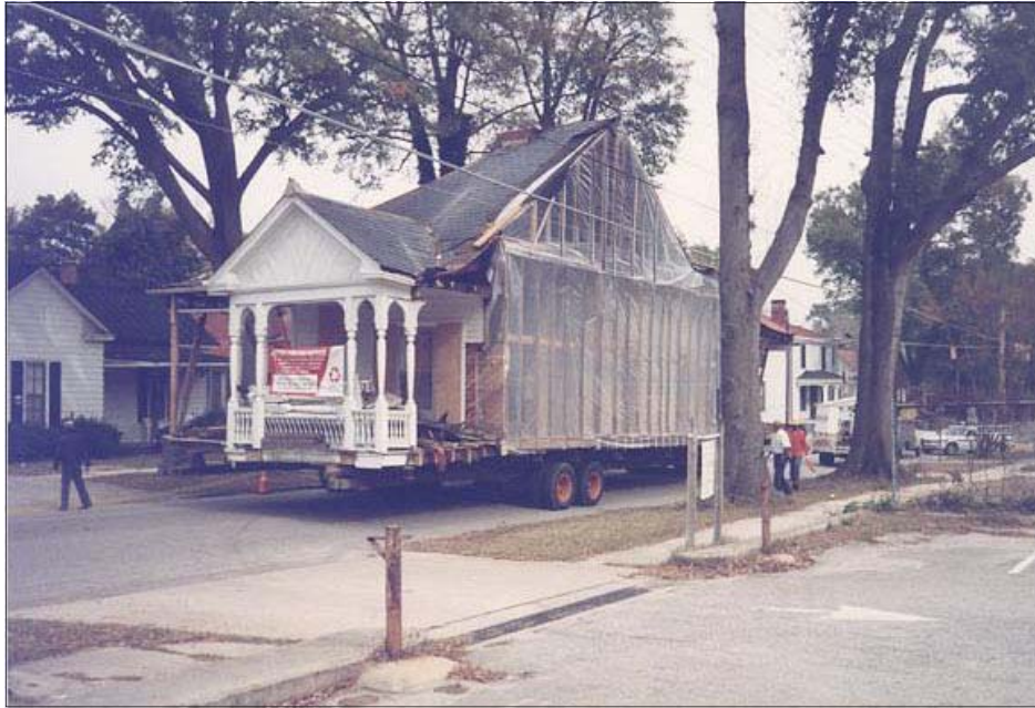
The McLaughlin House being moved in two sections. It is best to move the house in one unit, however the width of the house and street rendered that impossible in this case.
