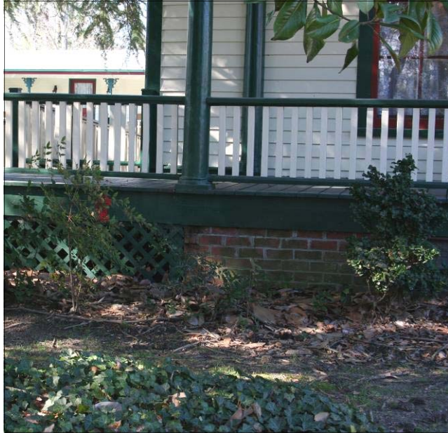
Example of lattice used to differentiate a new foundation from an original masonry foundation.
