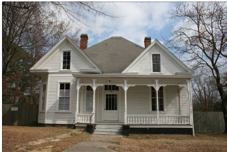
The wood spindle frieze, posts, brackets and balustrade are character-defining features of this wood home.
