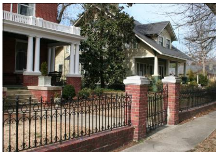
This brick pier and iron fence is another example of an historic fence treatment.
